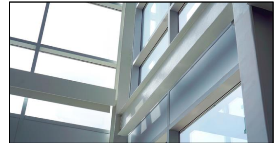
Great Northern Insulation Photo
