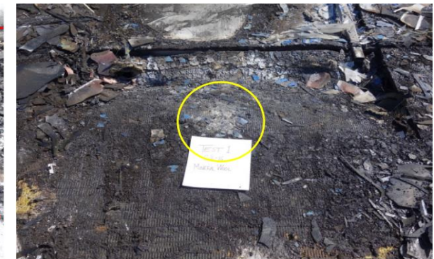
Yellow circle: Point of ignition without penetration of the mineral wool.
