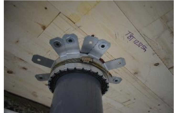
Exposed Side Before Fire Endurance
