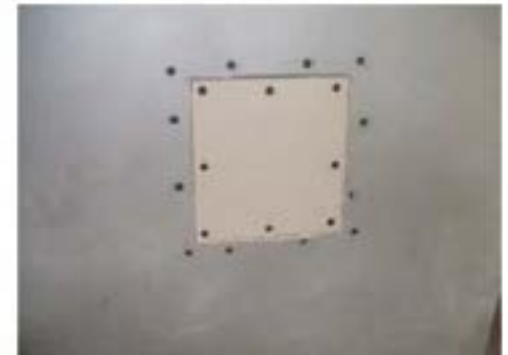
Figure 4: Apply Gypsum Panel Patch
