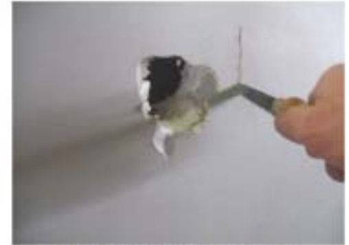
Figure 2: Square Off Damaged Area
