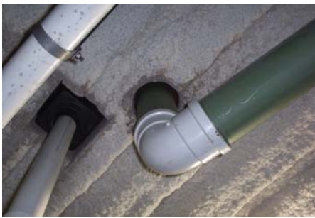
Prior to firestop system application.
