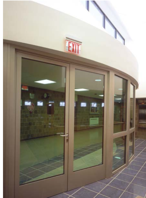
Glass ceramic has earned fire ratings up to 3 hours and can be specified in much larger sizes than wired glass.
