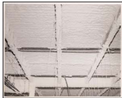
A Great Finished Deck
