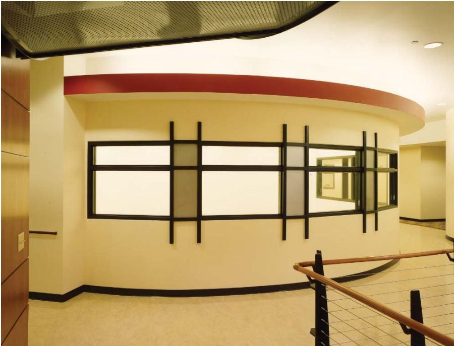
Another category of fire-rated glazing falls under the heading of glass fire walls.
