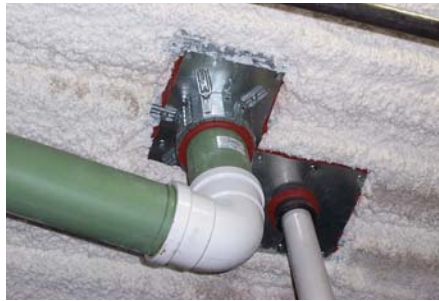
Penetrations protected with firestop system.
