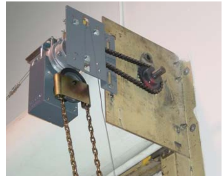
After retrofitting, a fire door has a simplified self-contained system with a release and governor integrated into the retrofit fire door operator.
