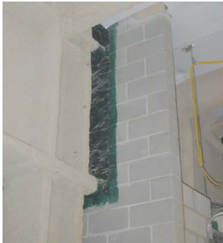
Fireproofed beam through block is shown.
