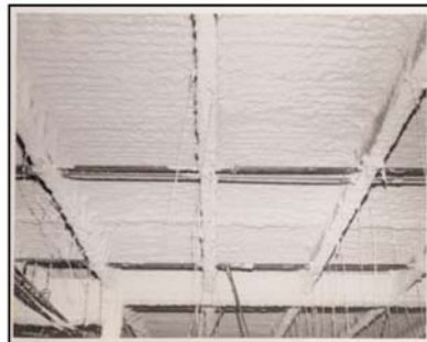
A Great Finished Deck
