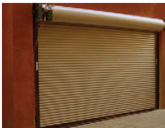
A rolling door is an effective method of compartmentation.
