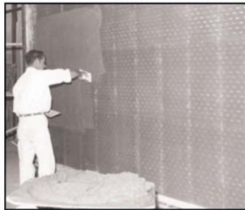
Fire Rated Walls
