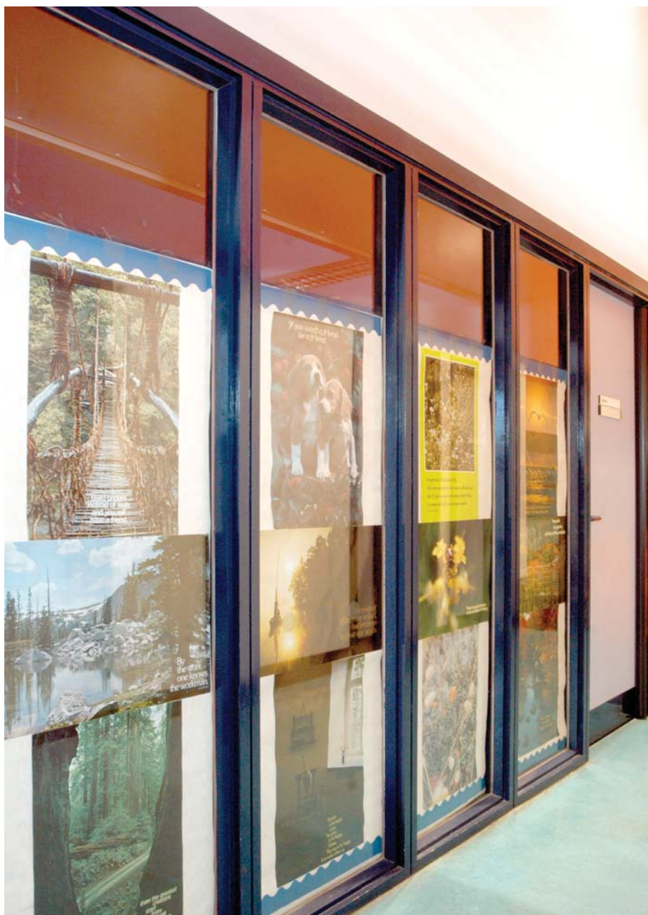
Fire glass protects compartmentation's integrity while allowing occupants to see what threat may be on the other side of the barrier.
