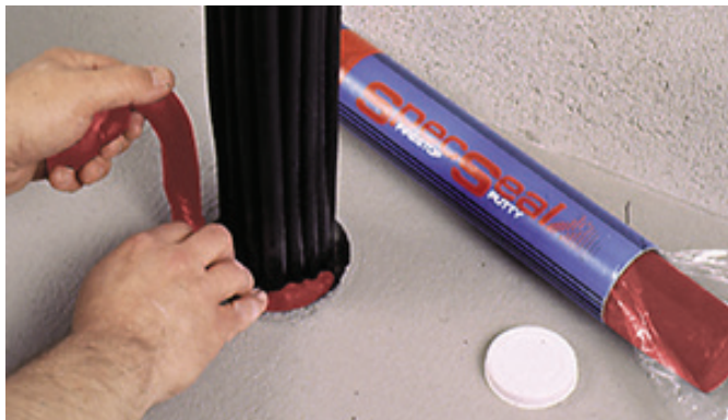
Figure 3 illustrates a typical malleable firestop putty that should be kept on hand for retrofittable applications. STI photo
