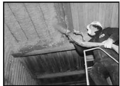
Applying the Proper Thickness
