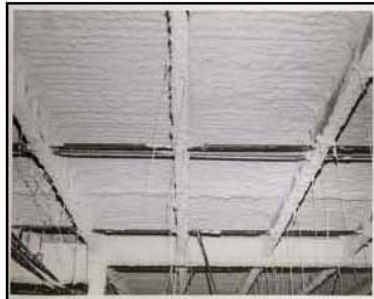
A Great Finished Deck
