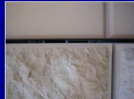
Exterior building materials sealed
