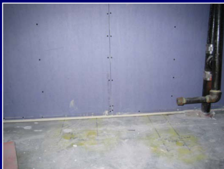
Wallboard off floor & sealed
