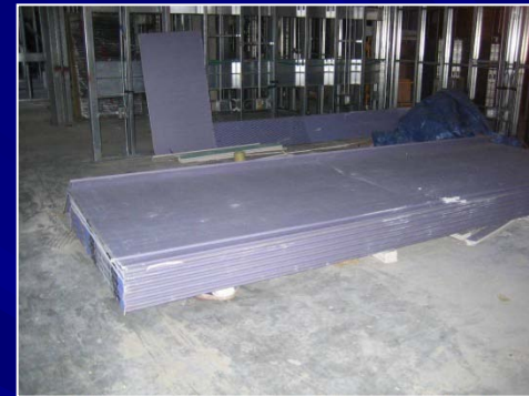
Storage off floor for water protection
