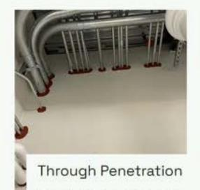
· A through penetration firestop is a system designed to prevent the spread of fire and smoke through openings in
