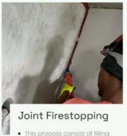
· This process consist of filling openings and joints between walls and floors with fire-
